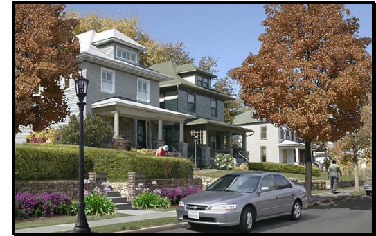
Traditional Neighborhood Development: Narrow setbacks, sidewalks and on street parking on neighborhood streets
