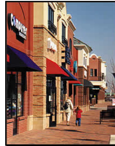
Detailed architecture on strip commercial facades
