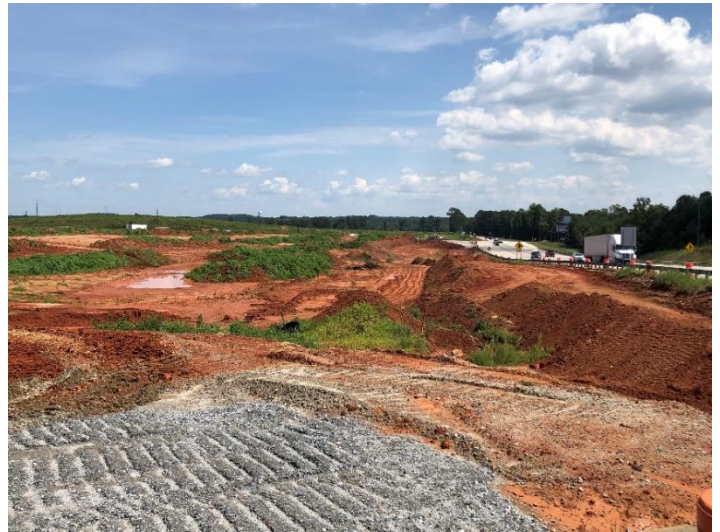
Figure 4: Rapid growth along I-75 in Butts County
