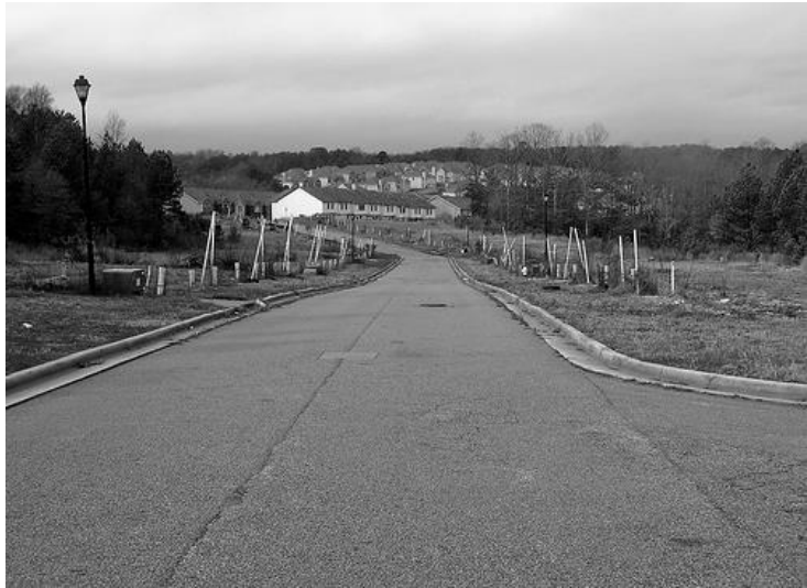
An example of an unfinished subdivision with protruding pipes.
