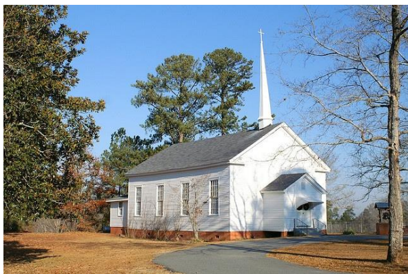
Although the original structure was burned during the Battle of Sunshine Church in 1864, the current Sunshine Methodist Church in Round Oak dates back to 1880.
