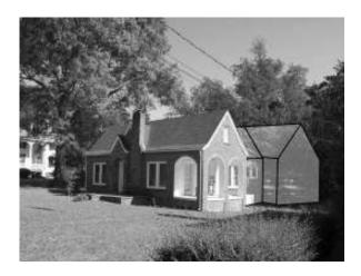
The proposed addition to this building is placed on the rear elevation, is clearly differentiated from the original structure, and is appropriately scaled.
