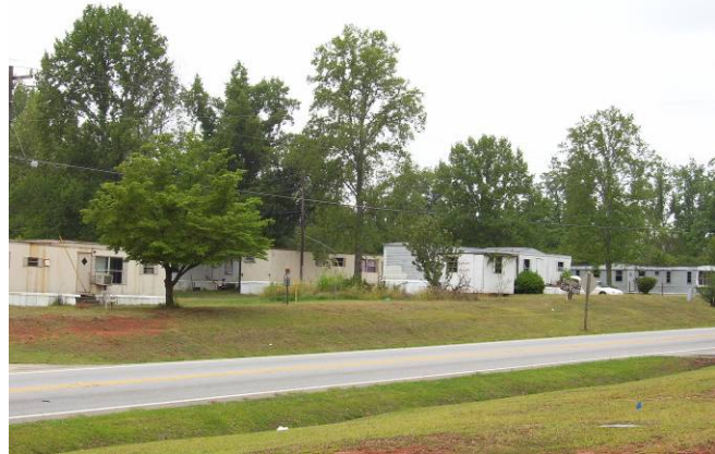
Mobile Home Park Along SR 36
