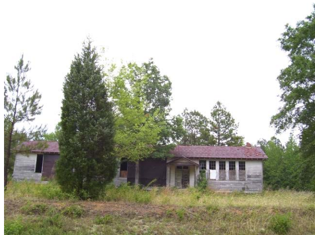
Historic Structure that Suffers from Neglect
