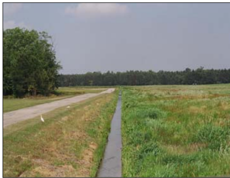
Sterling Creek Wastewater Treatment Facility constructed wetlands
