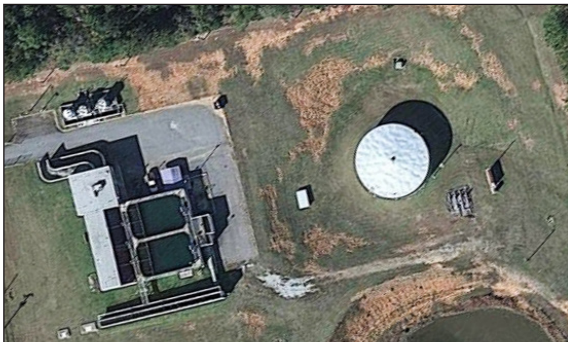
The Aonia Water Treatment Facility opened in 1978 and provided a capacity of 2 million gallons per day.
