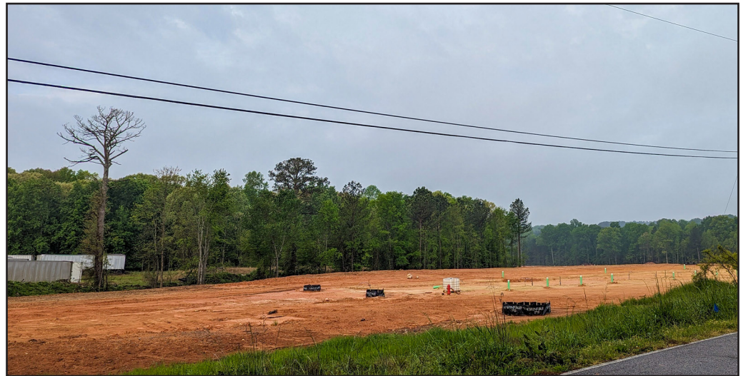
A new subdivision is under construction on Ashley Drive.
