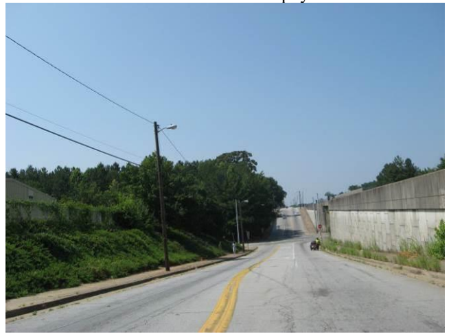
View south on Murphy Ave SW
