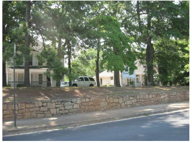
View of Subject from Murphy Ave SW
