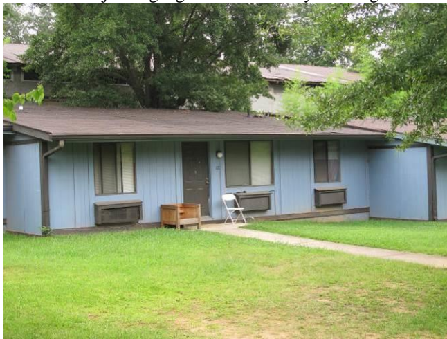
Subject one-story residential building
