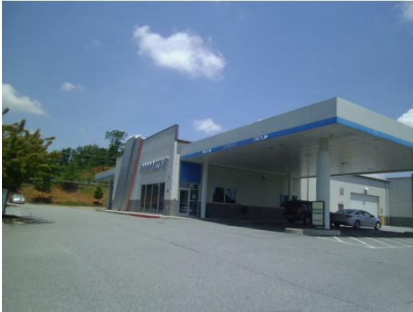
Progressive Auto Claims Center, south of site
