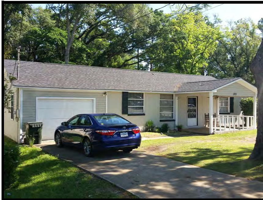
Typical single-family home southeast of site
