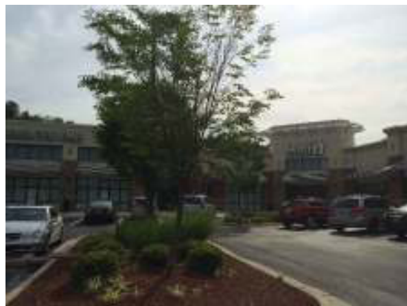
Kruti Plaza (shopping center) bordering the site to the southwest
