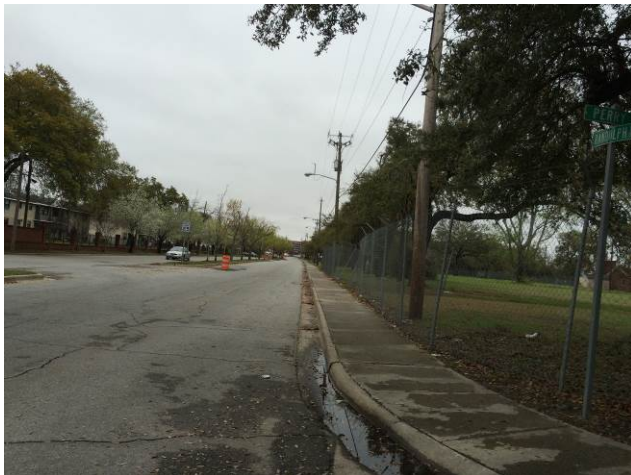
View north along Randolph Street
