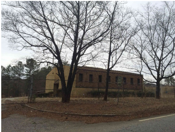
DeKalb County Department of Transportation facilities just northwest of the site
