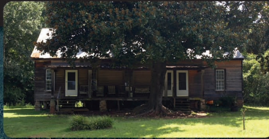
Historic Home, Monroe County
