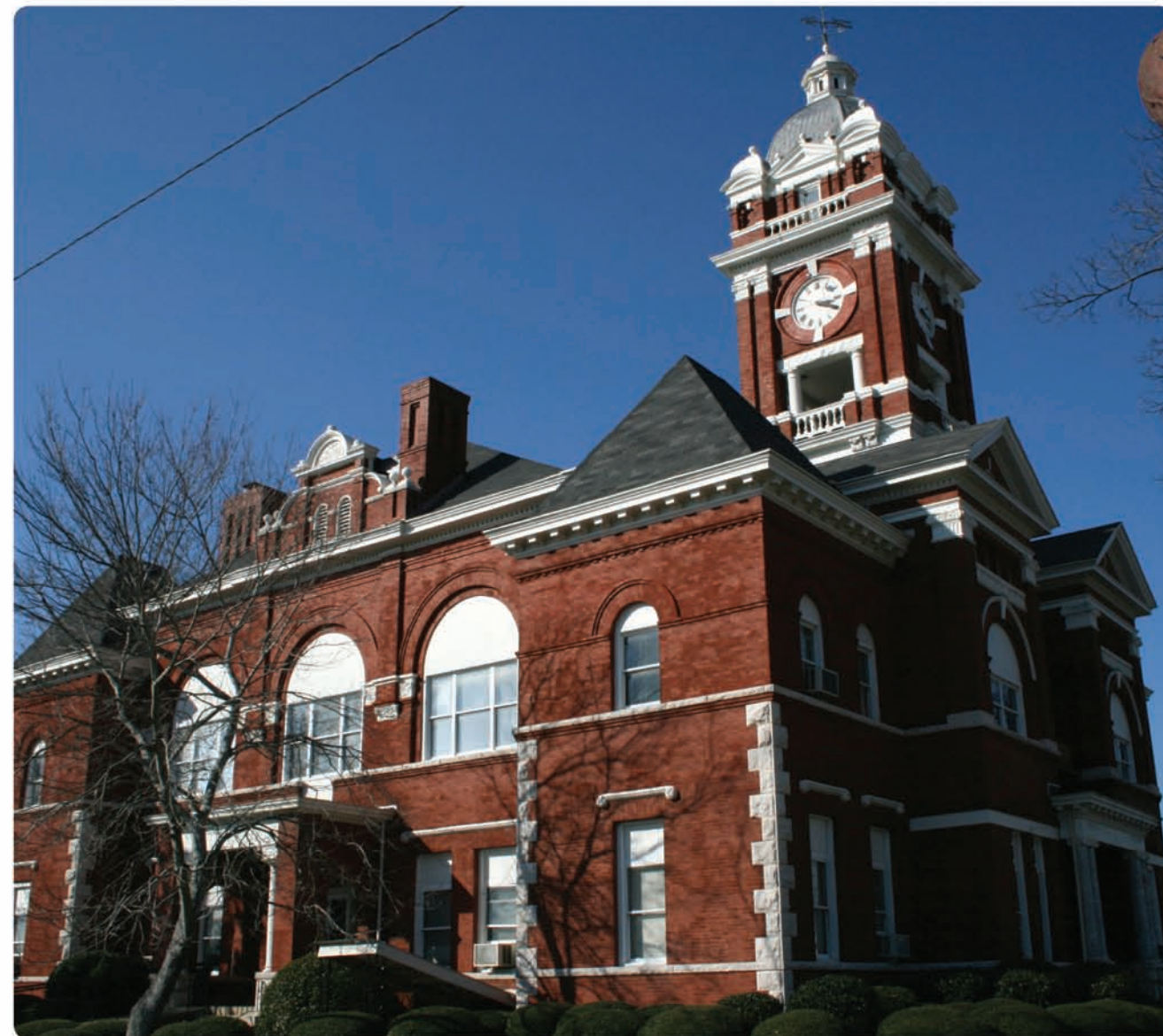
Monroe County Courthouse, Forsyth, 2010.
