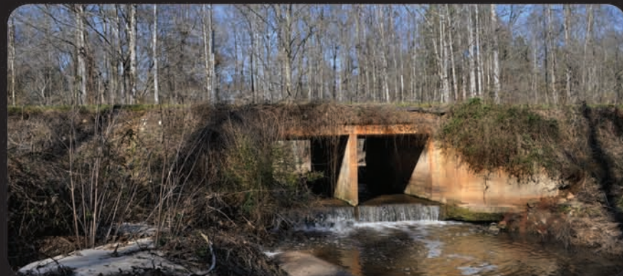
Cole Creek Culvert, Constructed 1939 , Lamar County
