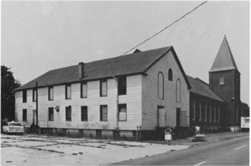
13. Springfield Baptist Church, Augusta, Richmond County. Constructed in 1801, enlarged in 1820, purchased and moved by the Springfield Baptist congregation in 1844. (James R. Lockhart for HPS)
