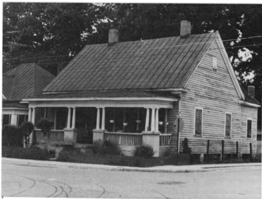
10. William McNatt House, Augusta, Richmond County. The ca. 1900 house built and owned by one of Augusta's foremost black builders. (Richard Dozier)
