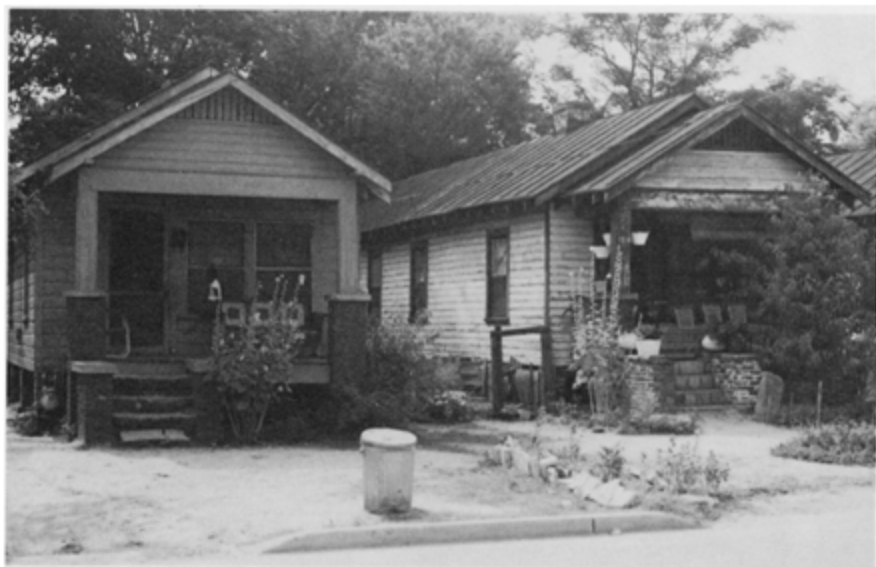
6. Early twentieth-century shotgun houses in the Bethlehem community of Augusta, Richmond County. (Richard Dozier)
