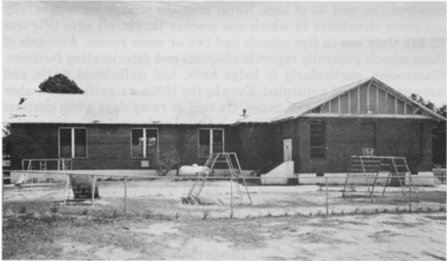
25. Lamson-Richardson School, Marshallville, Macon County. Constructed in 1915, rear gymnasium wing demolished in 1983. (James R. Lockhart for HPS)
