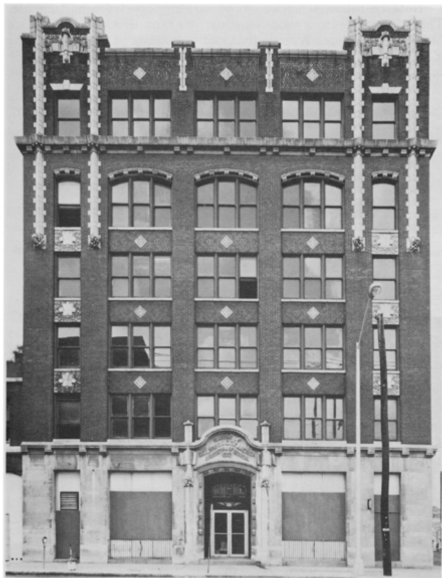
34. Odd Fellows Building, Atlanta, Fulton County. Constructed in 1912. (James R. Lockhart for HPS)
