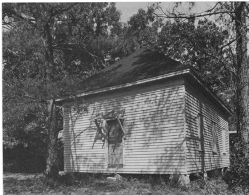
23. Chestnut Grove School, Athens vicinity, Clarke County. Constructed in 1896, an extant example of a rural one-room school for black children. (James R. Lockhart for HPS)
