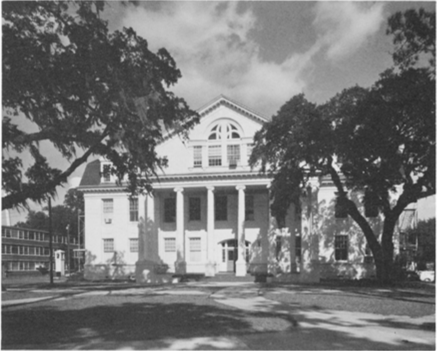
29. Hill Hall, Savannah State College, Savannah, Chatham County. Constructed in 1901 by students at the college. (James R. Lockhart for HPS)
