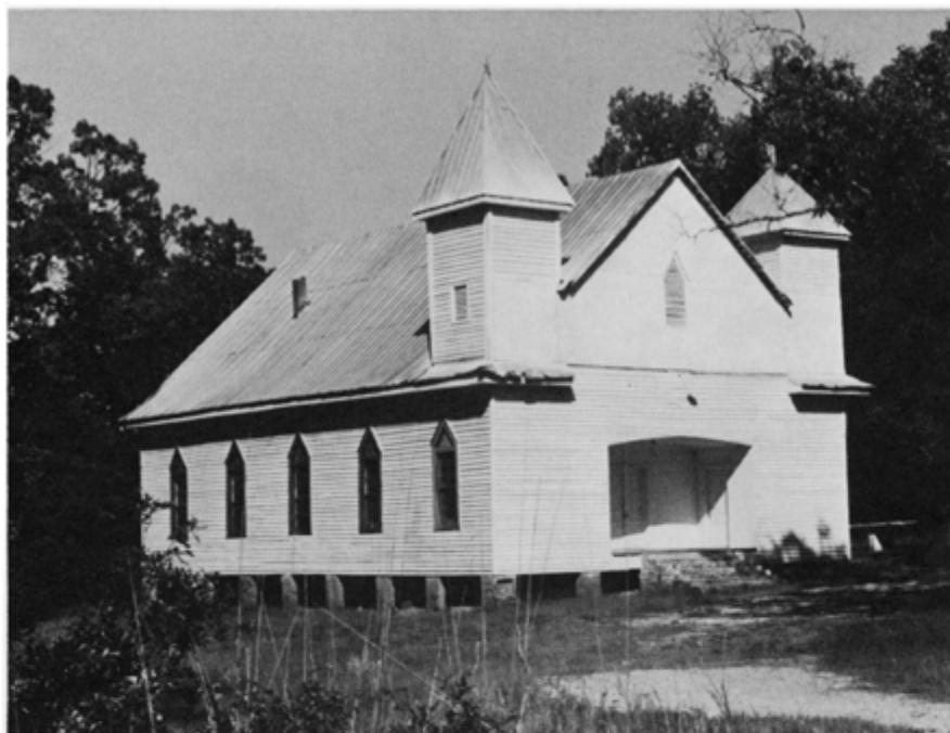
15. Church in rural Hancock County illustrating corner towers, central entrance, and weatherboard siding typically associated with rural black churches. (Richard Dozier)
