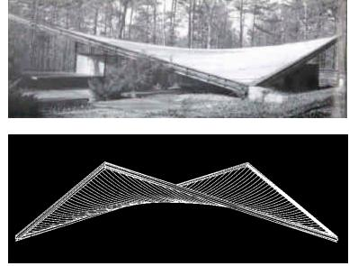
**Figure 16:** Ezra Meir-Catalano House, Raleigh, NC (1955) This is probably the best-known house of the North Carolina school. Catalano used a dramatic hyperbolic parabola roof form, anchored at two points, reminiscent of airplane design to create one of the best-known examples of roof architecture. The house also has the rare distinction of being publicly praised by Frank Lloyd Wright. Currently the house is for sale and in need of substantial restoration.
