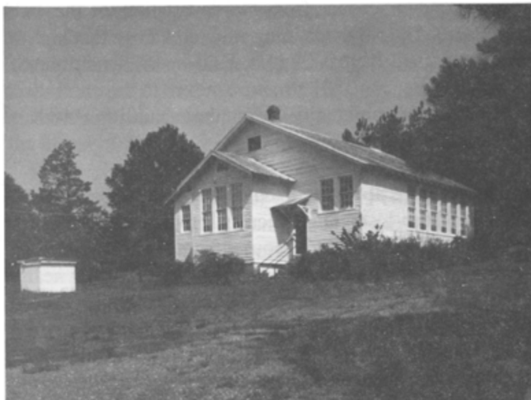
After Rehabilitation, Noble Hill School, Cassville
